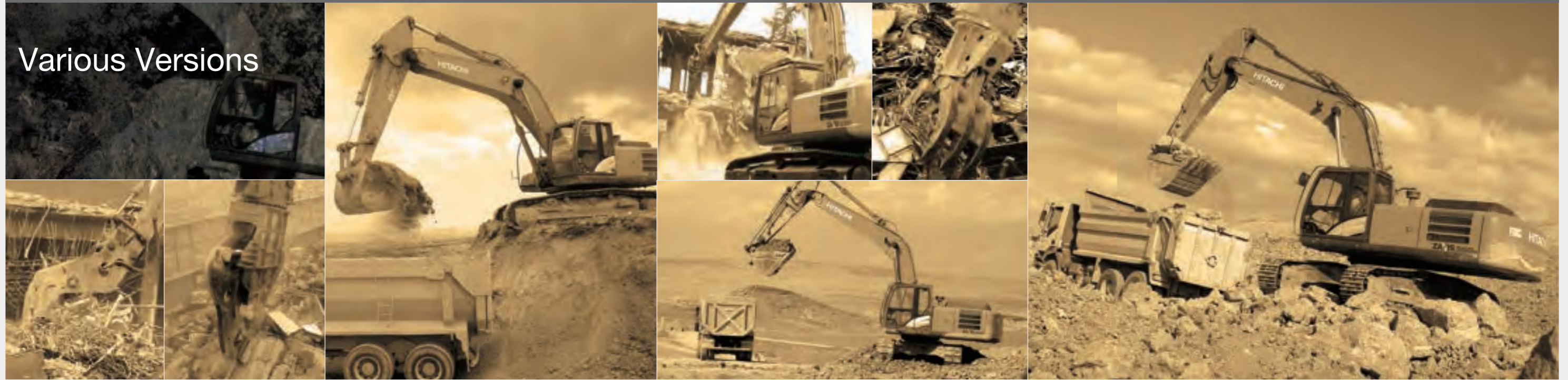
The photos above show machine images at work, which include machines other than ZAXIS 240 series.
